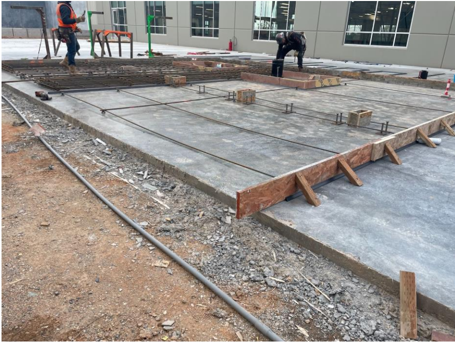
Tilt panels formed and placed
