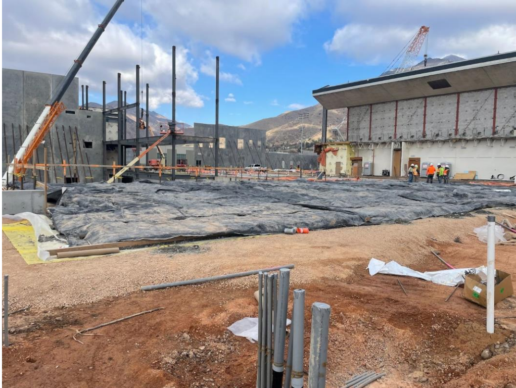
Administration area slab
