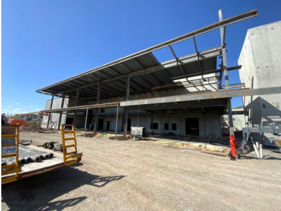
Canopy in front of the auditorium
