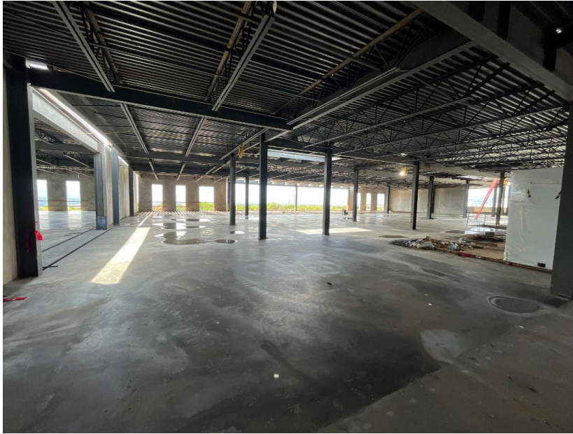
Slab placed at the chemistry labs as well as a few of the general classrooms
