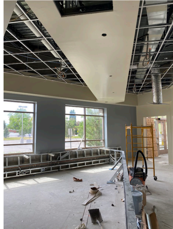
Ceiling grid installed
