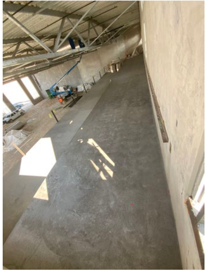
Concrete has been placed in spectator seating area
