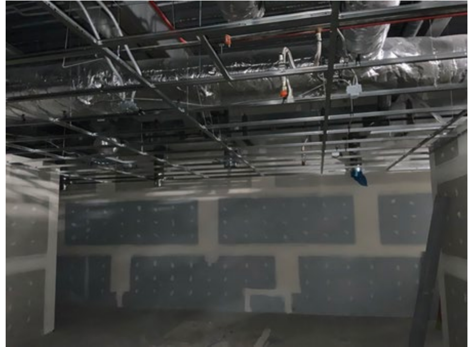
Drywall installed on the first level
