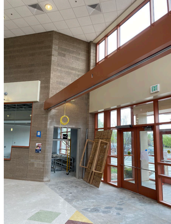
Beam has been painted
