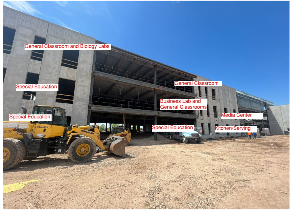
View of the main academics building from the future courtyard
