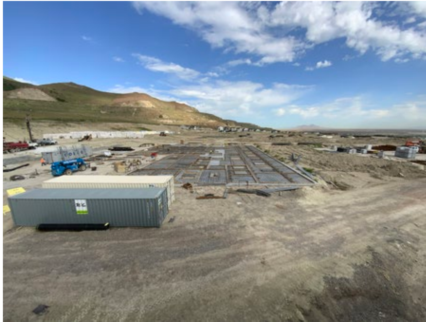
Tilt panels being prepared for concrete
