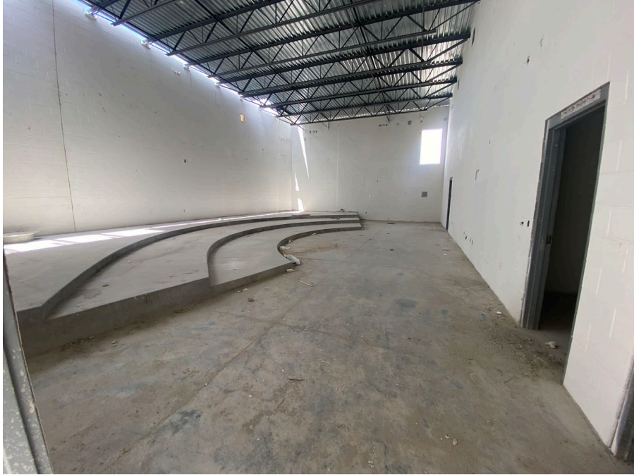
Choir room in progress
