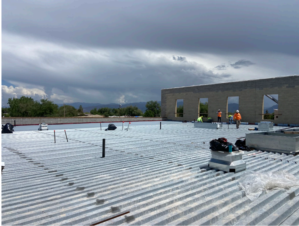
Roof decking in place over kitchen
