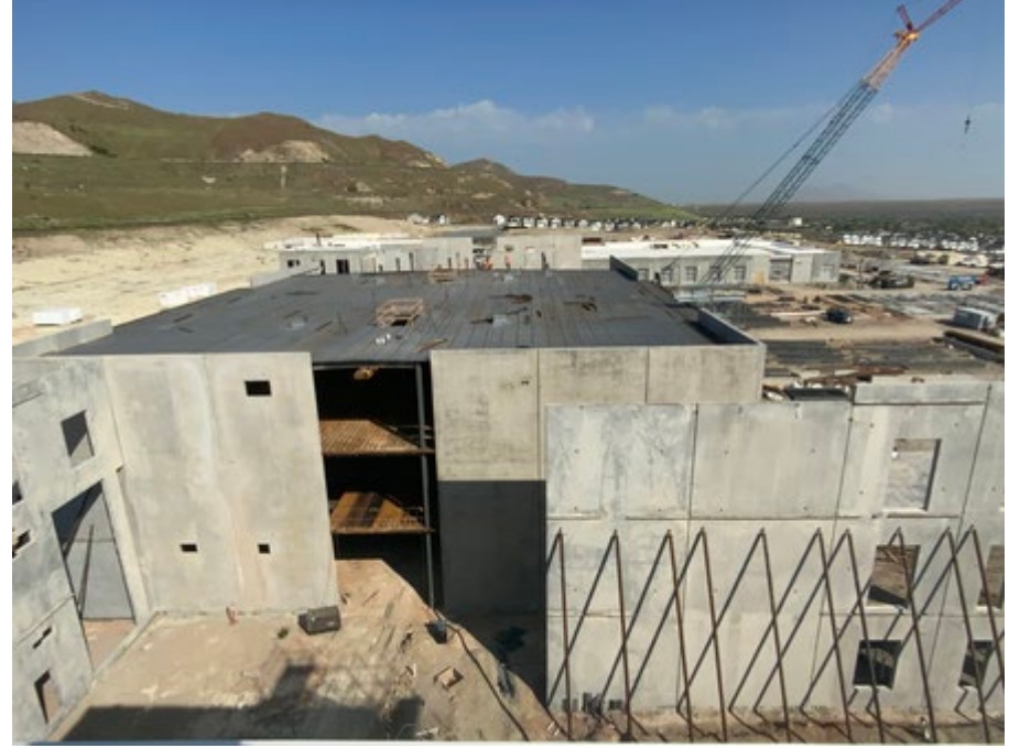
Decking continues to be placed in arts area
