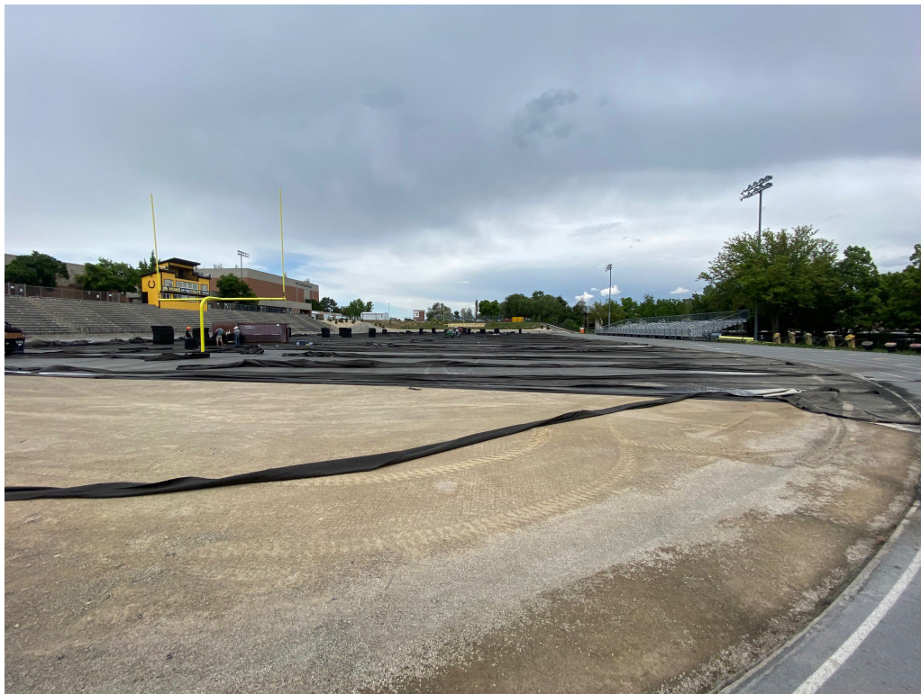
Exposing existing subgrade
