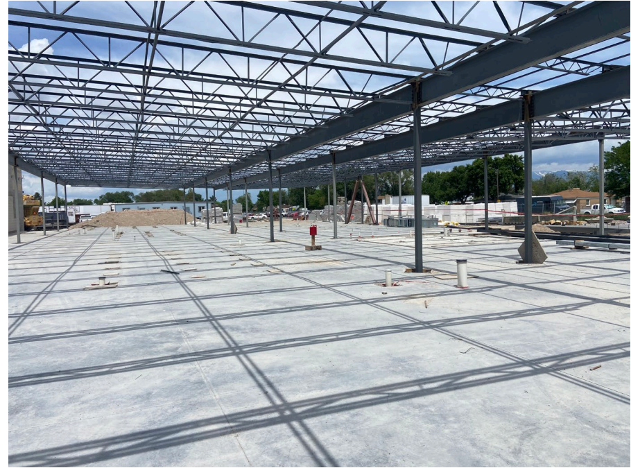
Steel over CTE area
