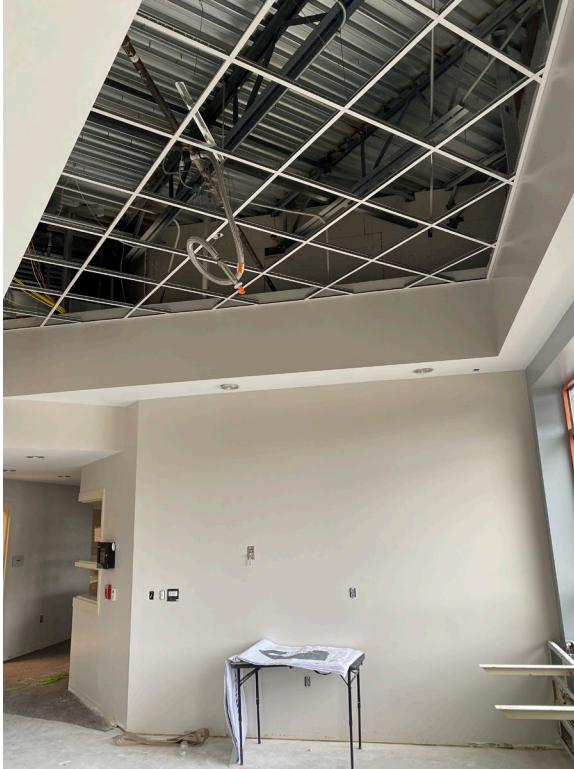
Ceiling grid is installed
