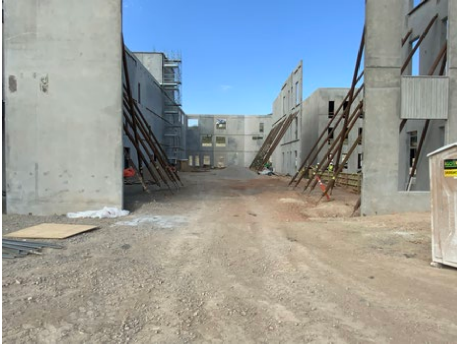
Academics walls have been set and braced
