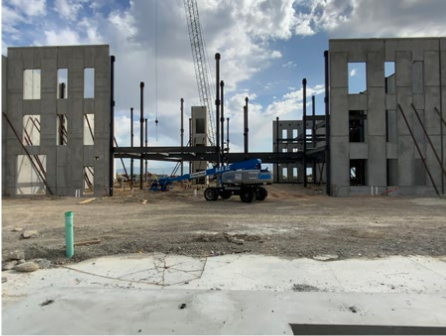
Steel structure being raised in the mechanical and academics area
