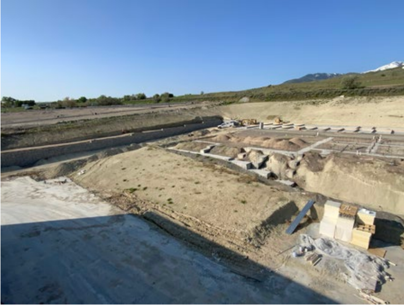
Retaining wall on south side of the building
