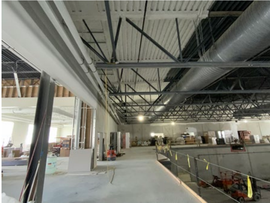
Painting and insulation on second level of gymnasium
