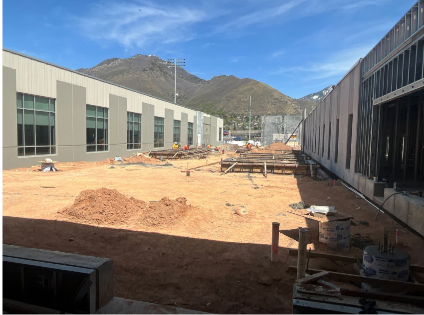
Courtyard prepared for concrete
