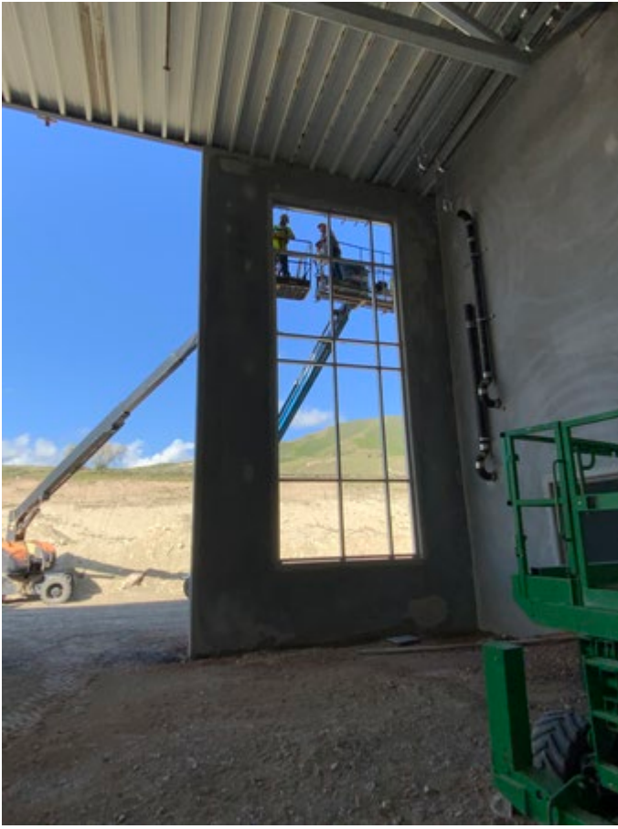
Aluminum frame for curtain wall in pool
