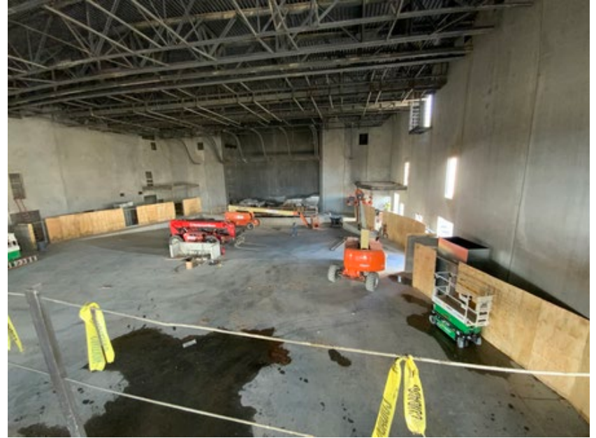
Cast-in-place walls and storage area in auditorium
