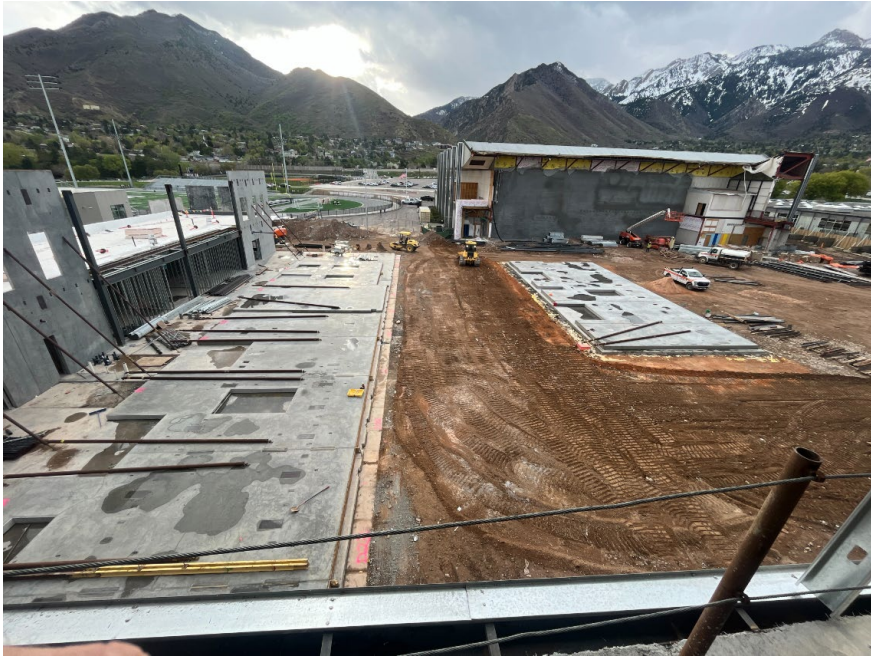
Tilt panels for the south half of the administration suite placed, while part of the cafeteria slab has been placed
