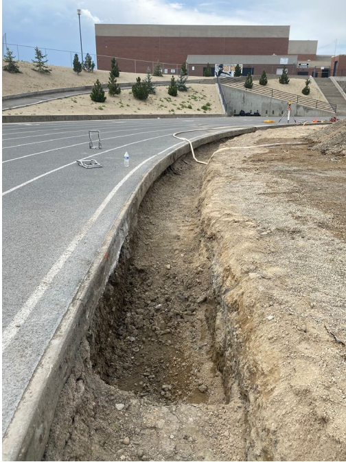
Removal of old drainage system
