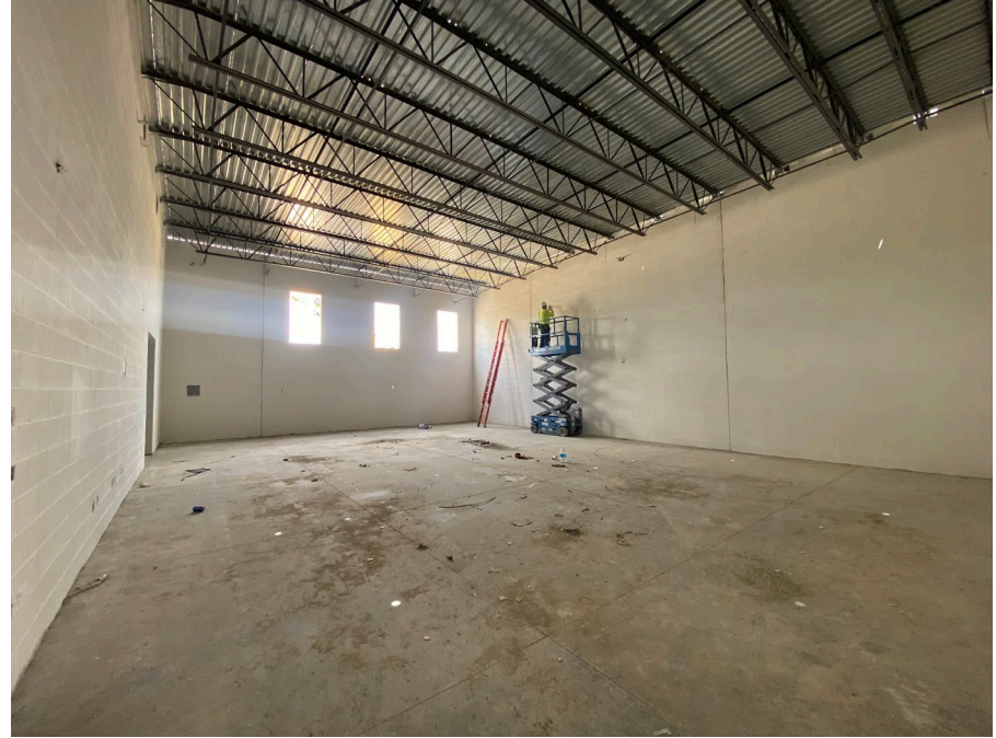
Band room in progress
