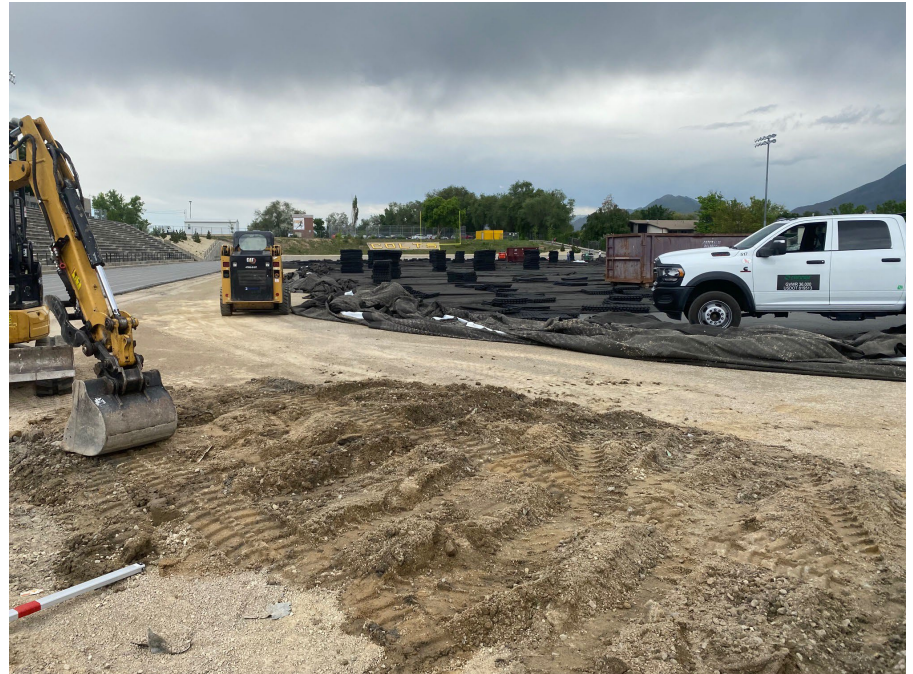
Turf removal and surface preparation
