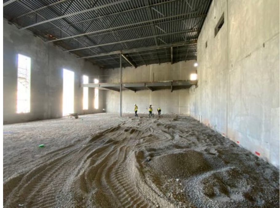
Backfill in the band/orchestra area
